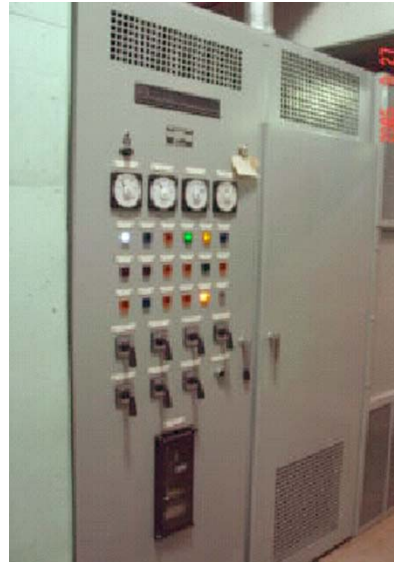
Figure 3 - Basler Static Shunt Exciter
