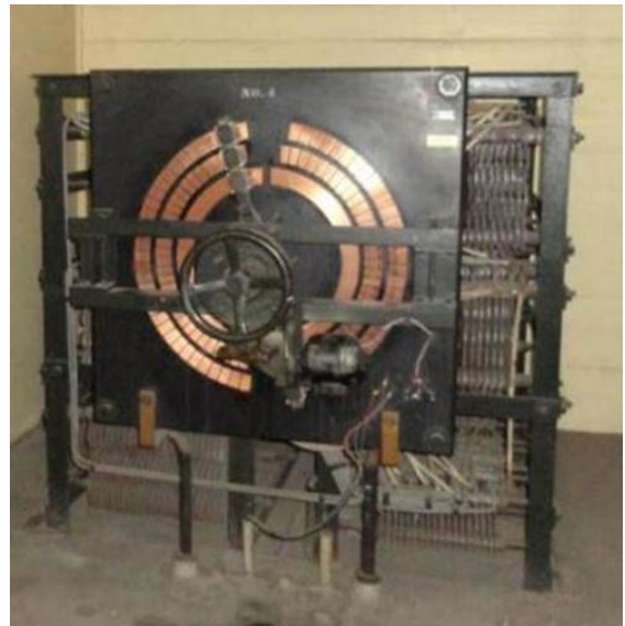
Fig. 1 1940's voltage adjust rheostat
