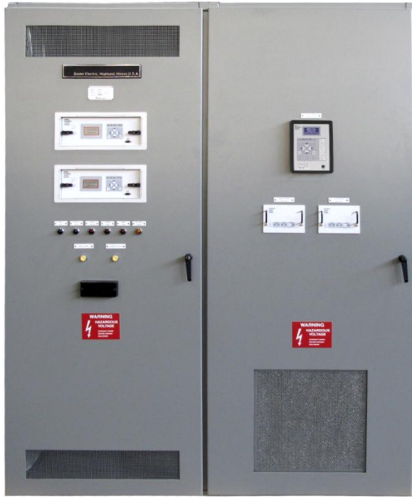
Fig. 13 Complete static exciter cabinet less the PPT
