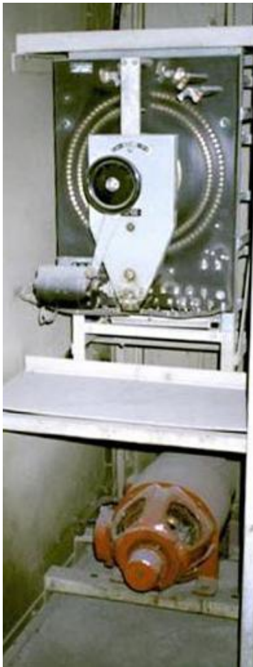
Fig. 3(B) Amplidyne voltage regulator
