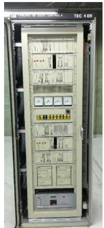
Figure 2. Unitrol M System Cabinet
