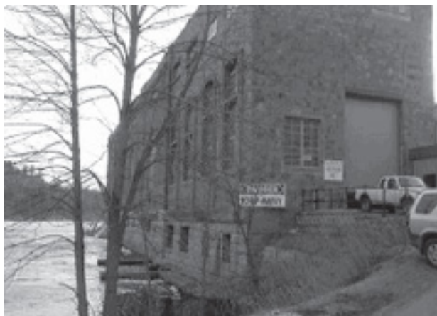
Figure 2. At facilities with slow speed hydros, like the one above, there can be tuning challenges without negative field forcing voltage regulators.
