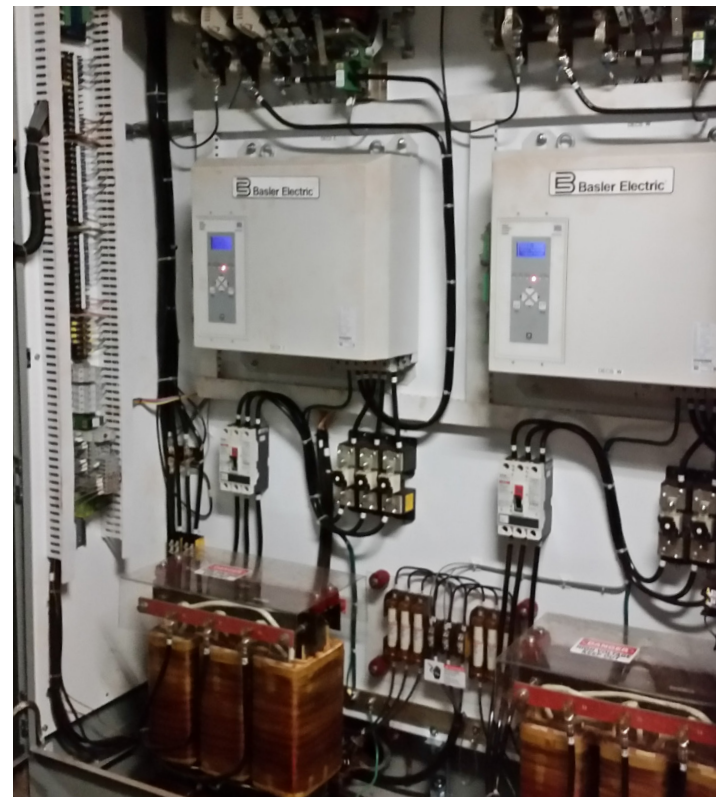
Figure 4b. DECS-250E with Field Application Device
