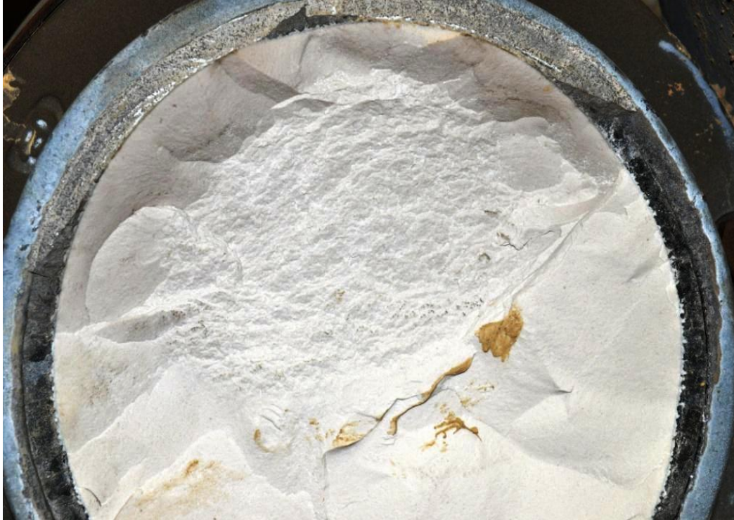
Fig. 4 – Bus Insulator Fracture [1]
