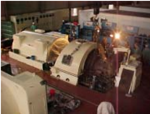
Fig. 2: Turbine Generator Undergoing Inspection and Test Prior to Purchase
