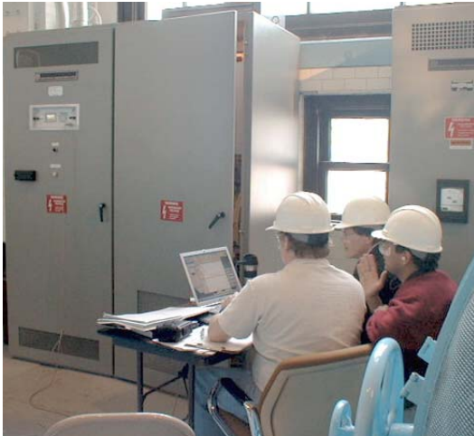
Figure 2: Laptop computers are connected into the excitation system serial port to gather information
