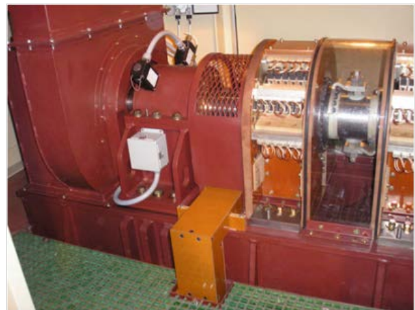
Fig. 7 New Slip Ring and Brushes
