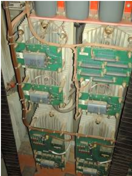
Figure 2: Existing 3 SCR, 3 Diode Half-Wave Bridge
