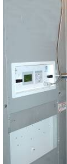
Figure 4: DECS-400 Installed in Cabinet Door
