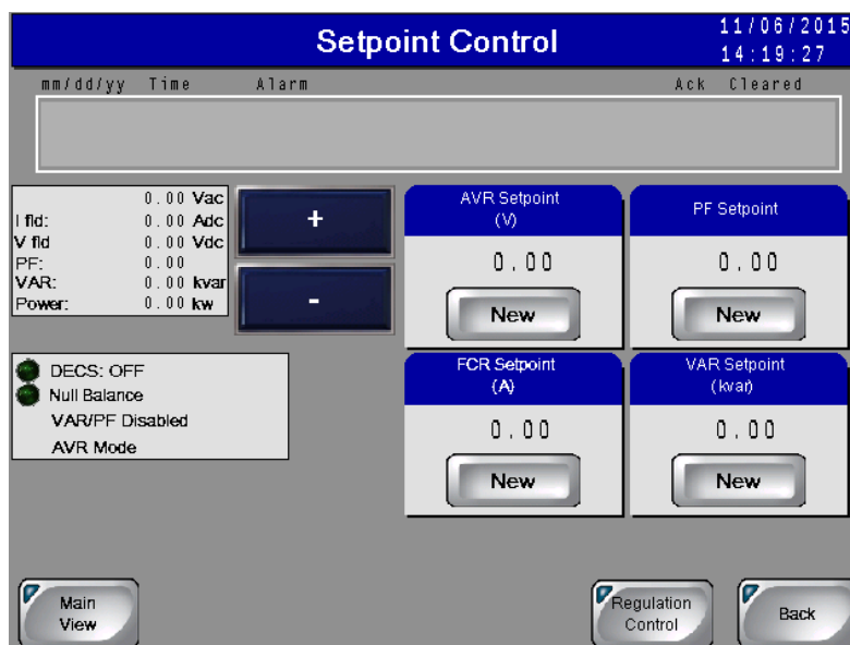
Figure 5-23. Setpoint Control Screen
