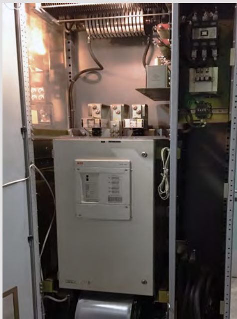
DC cable (aux section for cables in dark area) vs new DC bus stabs and cabling (improved visibility)
