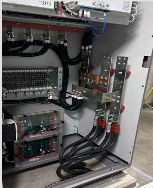
DC cable (aux section for cables in dark area) vs new DC bus stabs and cabling (improved visibility)
